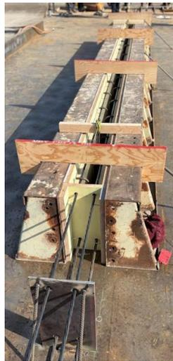
Figure 8: Formwork with stirrups and prestressing strands
