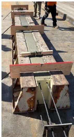
*Figure 19: Beam after concrete poured*
