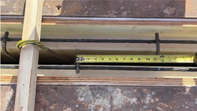
Figure 14 (right): Single lifting loop identifying side with 11 in. stirrup spacing
